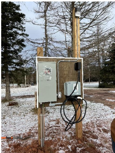
Figure 5-2: At-home charging solution demonstrated in Prince Edward Island (Photo Credit: PEI)
