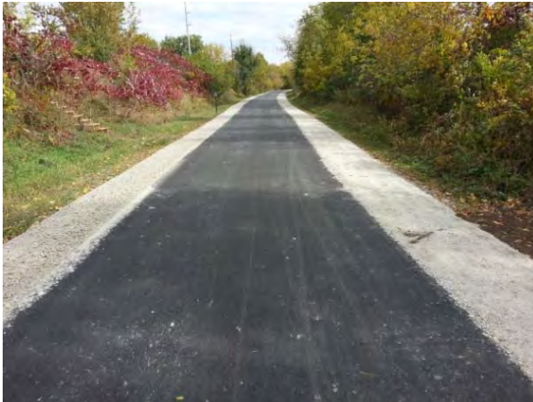
3m Asphalt Surface with 1m Gravel Shoulders Lindale Trail (Cedar Rapids, IA) [Source: linncountytrails.org]
