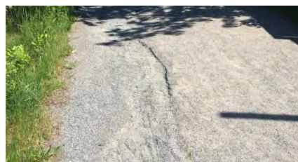
Rutting on Steep Sections
