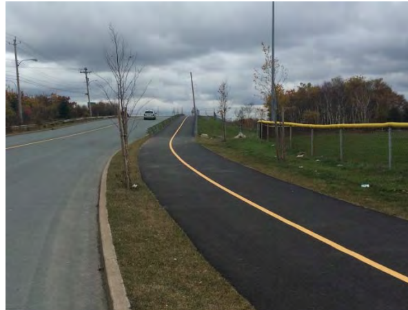
3m Asphalt Surface Greenway Highfield Park Drive (Dartmouth, NS)
