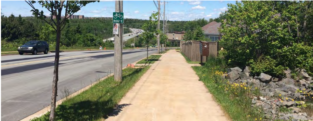
The existing 2.8-3.0m sidewalk could be widened into the grass boulevard to create a 4.0m wide surface
