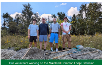
Our volunteers working on the Mainland Common Loop Extension.
