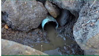
The piping installed.
