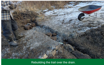
Rebuilding the trail over the drain.
