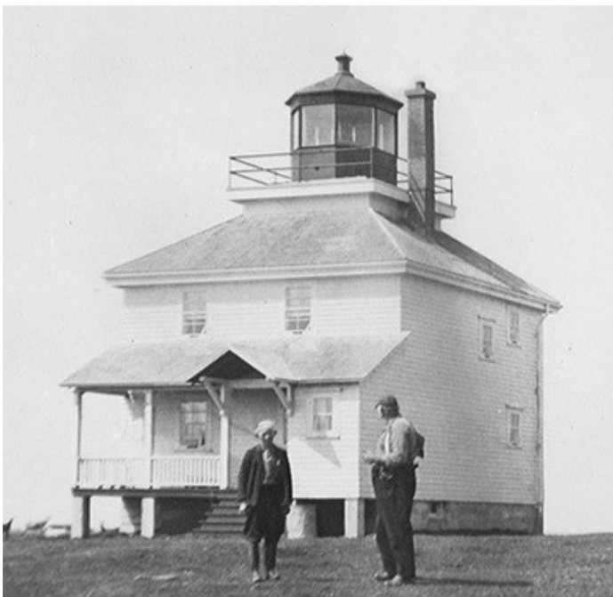
2 nd Pearl Island Lighthouse looked like this built same year Credit: Nova Scotia Archives
