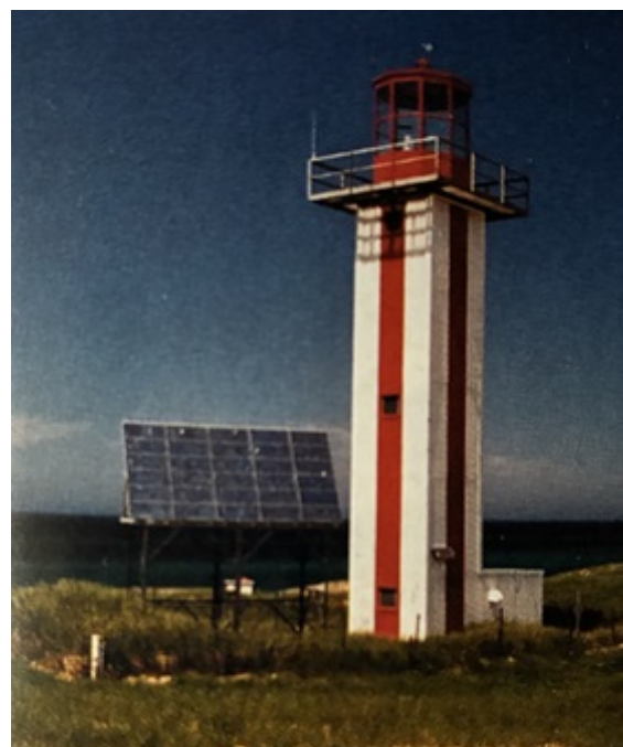
3 rd East End lighthouse Credit: Rip Irwin
