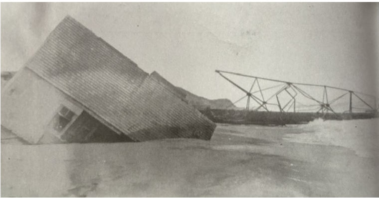
Old West End Lighthouse toppled by shifting sand Credit: Library and Archives Canada
