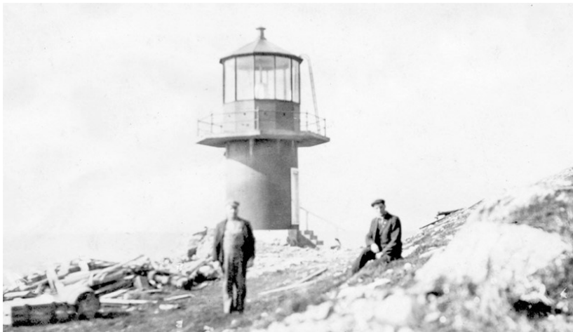
St Paul Island South Point (2 nd lighthouse on site) Credit: NS Archives
