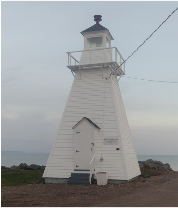
Spencer's Island Lighthouse Credit: Matthew Burke
