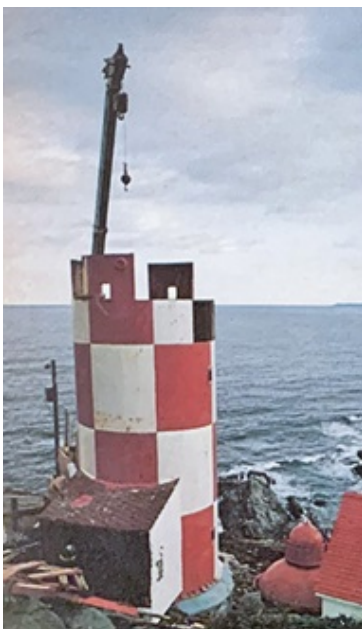
Dismantling Cape North Lighthouse 1980 Credit: Canadian Coast Guard
