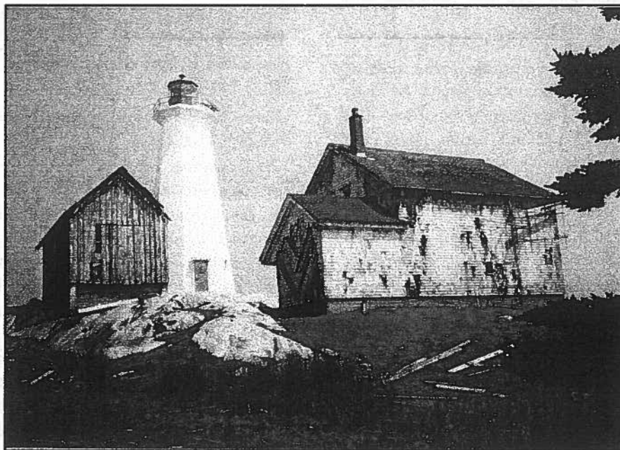
Neglected outbuildings surround the 1960 lighthouse at Cape Roseway. Nancy Eisener
