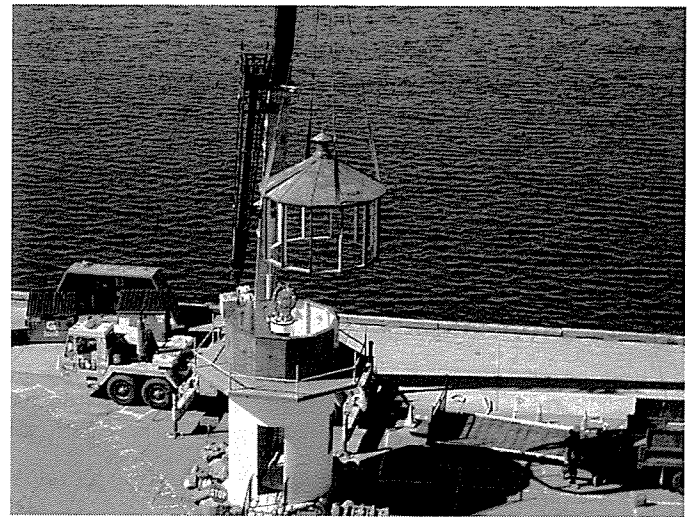
REMOVING THE LANTERN. DFO/COAST GUARD
