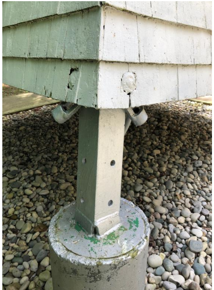
Stokes Bay Rear Range tie cross bracing brackets
