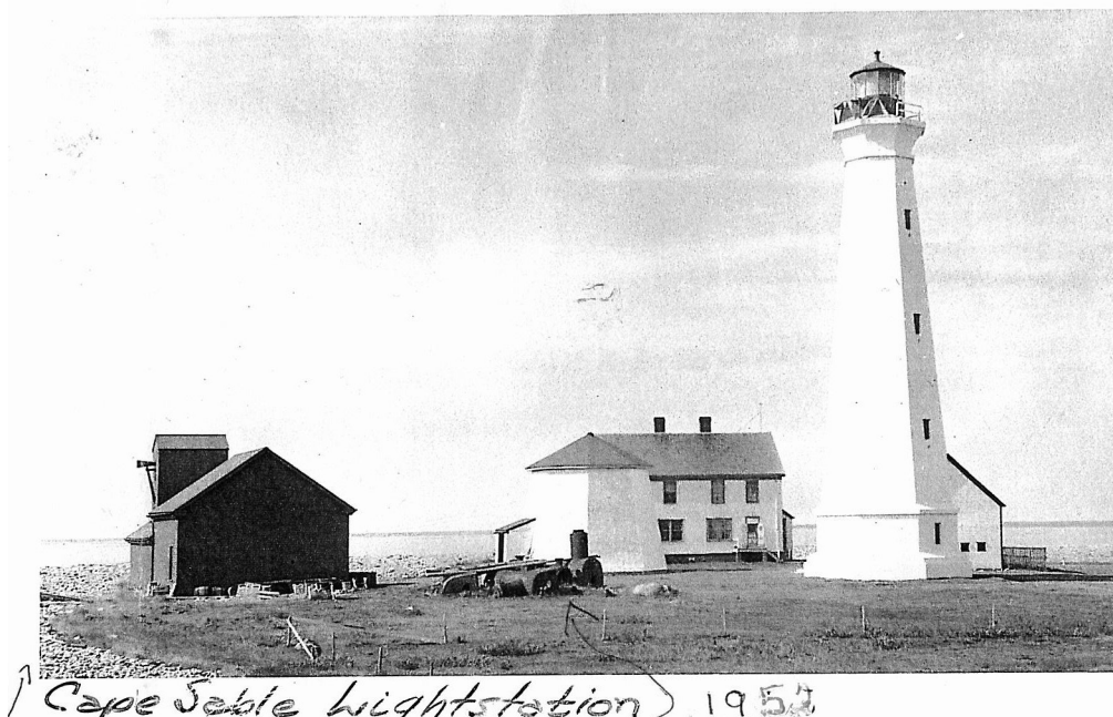
Cape Sable Light and Fog Alarm Station, 1952, from the east. Left to right: Fog Alarm building; old steam boilers; Old Light, shortened and used for storage; duplex dwelling; New Light, with radar reflectors on deck railing; barn. ·
