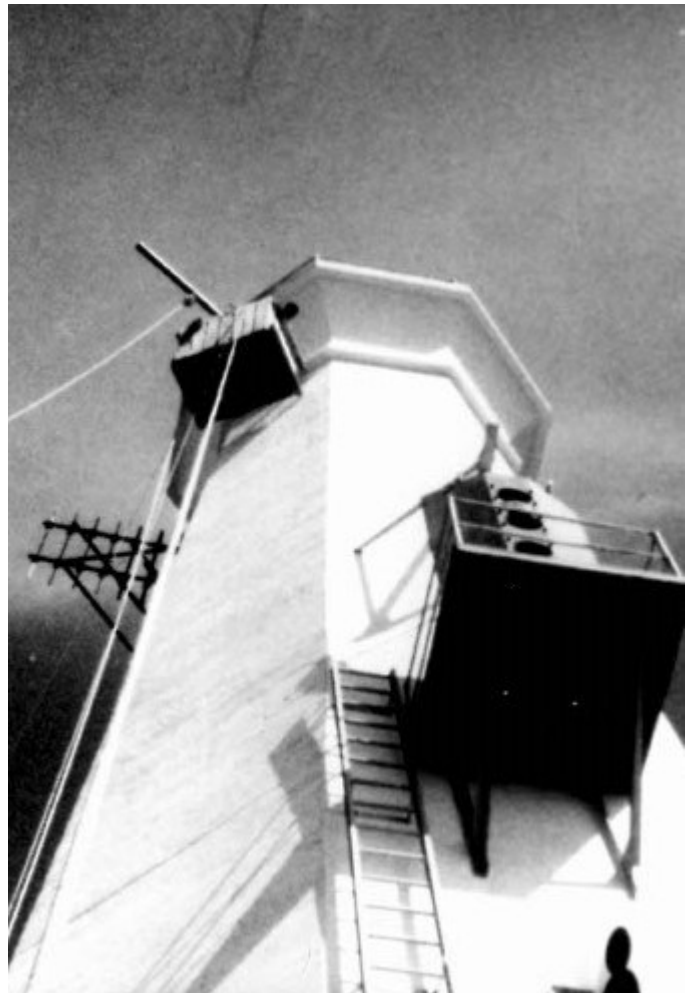
The Painting Box at the very highest point; circa 1978. At left, UHF radio antenna for communication with Yarmouth Marine Radio. Mid right, rack of 4 AGA electric horns; lower right, outside extensions of fog detection unit.
