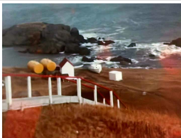
Staircase to Green Island Lighthouse.
