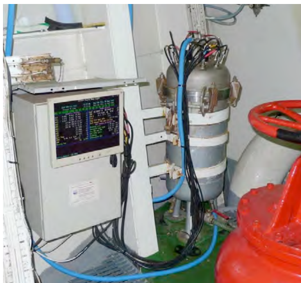
Figure 2.1. The SNOMS flow through tank and data unit installed on the MV Pacific Celebes , in the ship's machinery space.
